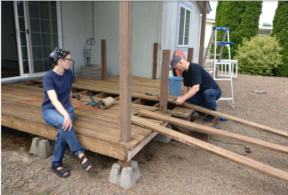
Working on deck repairs with our daughter, Nancy.
